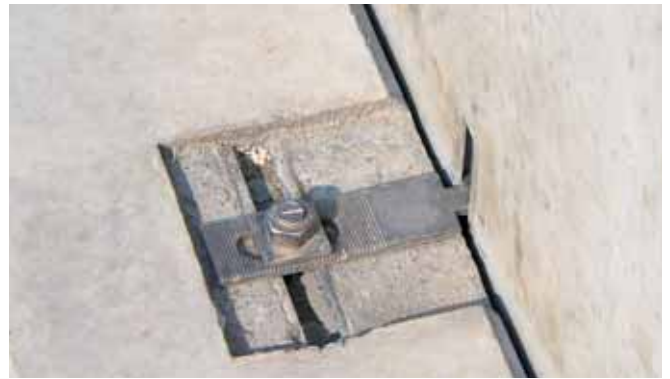
HALFEN HKZ Restraint tie with serrated washer
