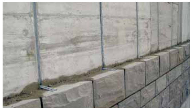
HALFEN ML Brick-ties anchor system
