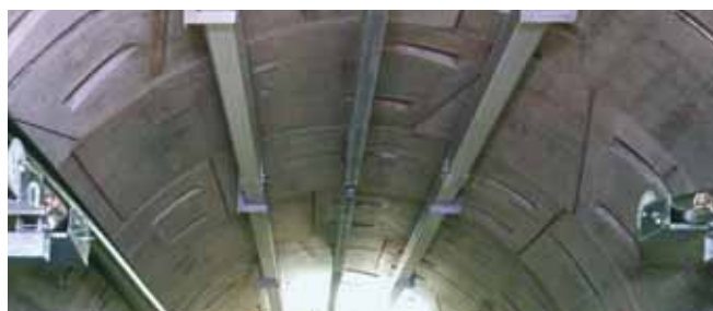
Curved HALFEN Cast-in channels in tunnel segments
