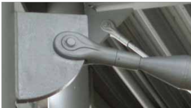
Compression system connected to a plate
