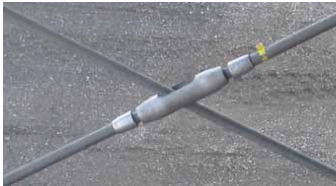
Cross-bracing with a cross-coupler
