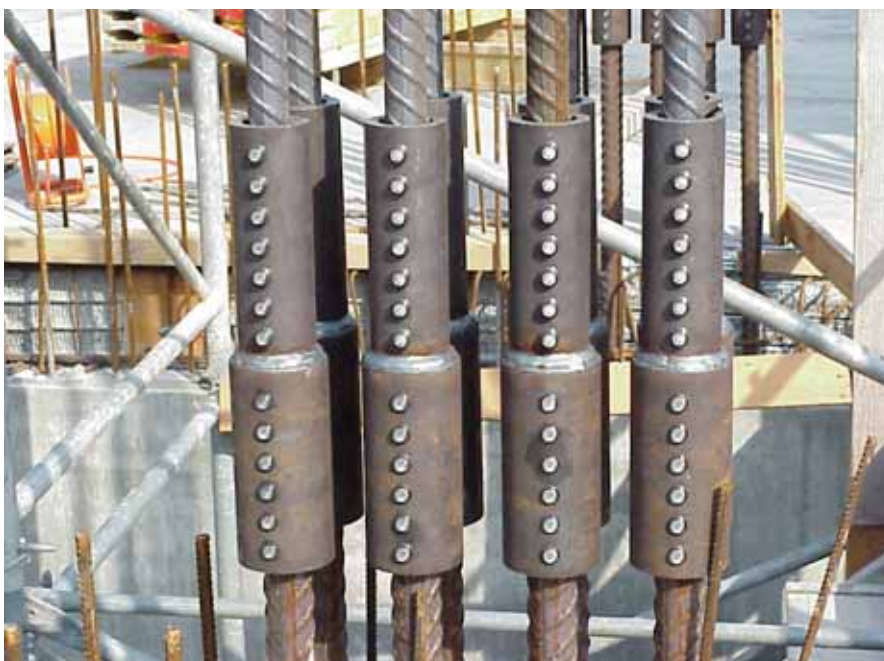
Support column with transition couplers
