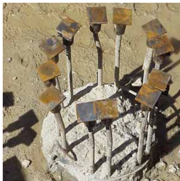
End zone detail in one pile
