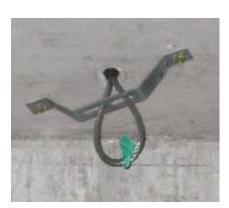
Cable loop installed in a lift head
