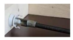
Press the identification cap on to the sleeve. The sleeve protection is in place on delivery.
