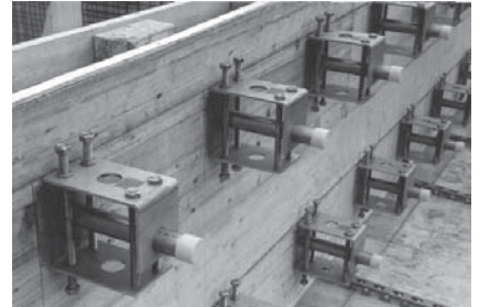
HSD-CRET sliding sockets nailed onto the formwork
