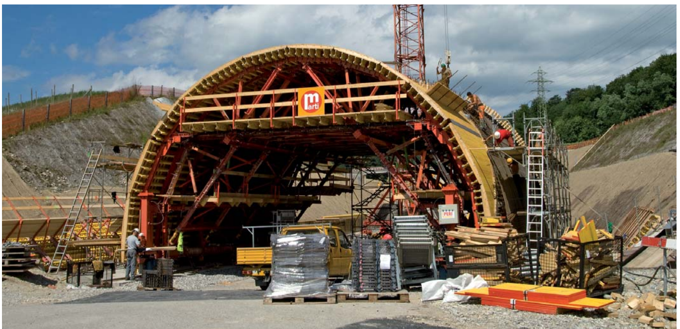
Application sample: HTA-CS on carriage mobile formwork
