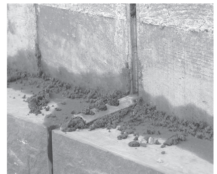
ML/BL Masonry connection
