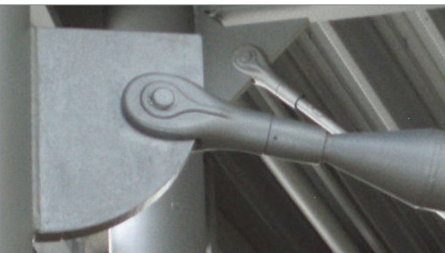
Compression system connected to a welded plate
