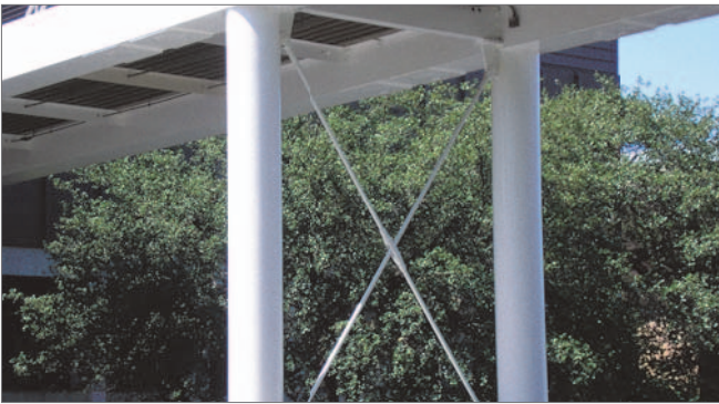
Cross-bracing with a cross coupler
