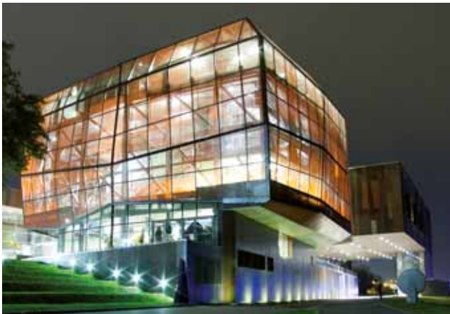
Kopernikus Science centre, Warsaw, Poland
