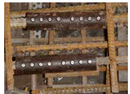
Join of a longitudinal reinforcement using standard couplers
