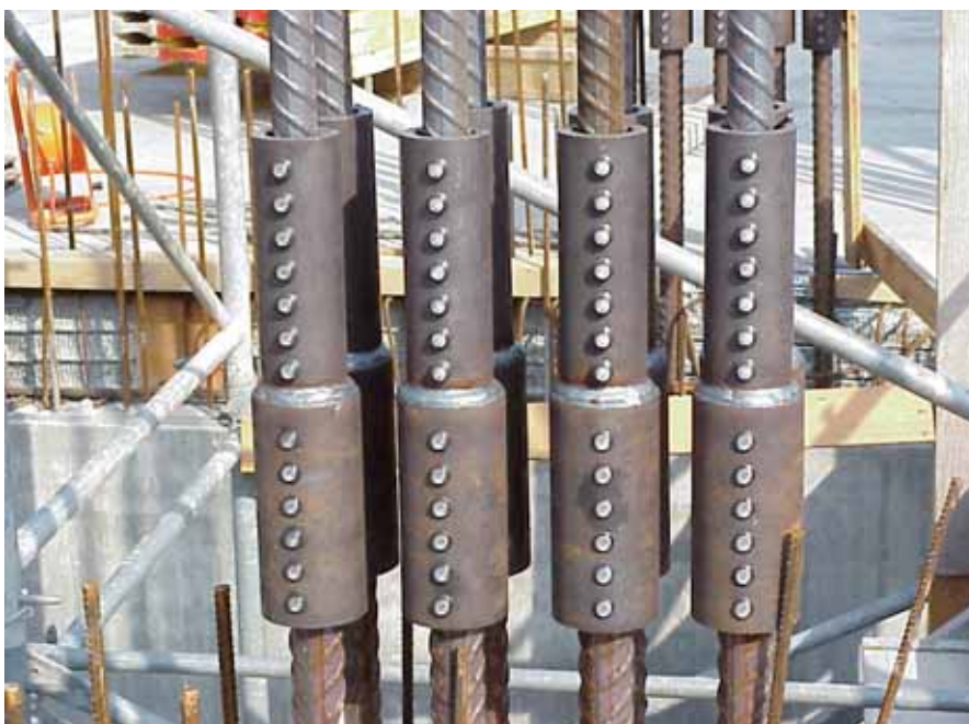
Support column with transition couplers
