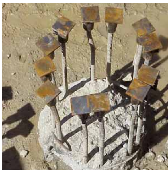
End zone detail in one pile
