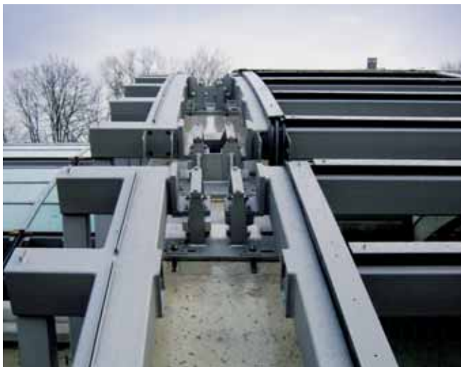
HZM38/23 channels in A4 steel used to attach the support structure of the steel roof to the top of the precast concrete roof beams
