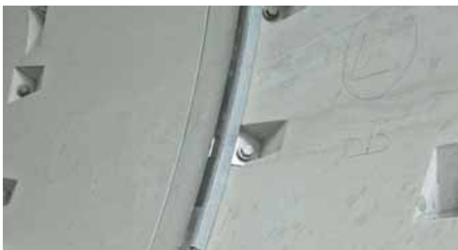
HM 72/48 Framing channel bolted to transverse joint
