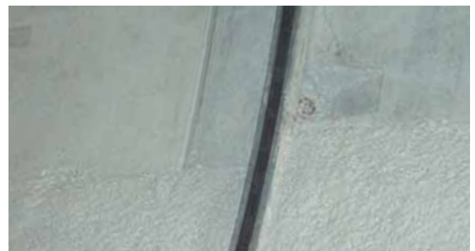
Tunnel wall with additional fire protection layer between the framing channels.
