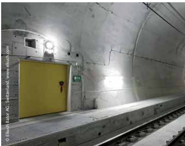
Cross passage door, closed, Lötschberg Base Tunnel
