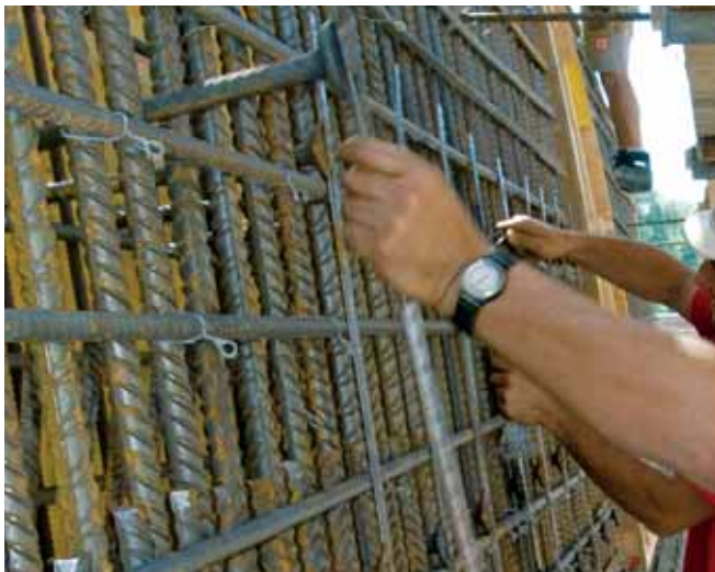
Fixing the HDB element in the reinforcement for the tunnel shell
