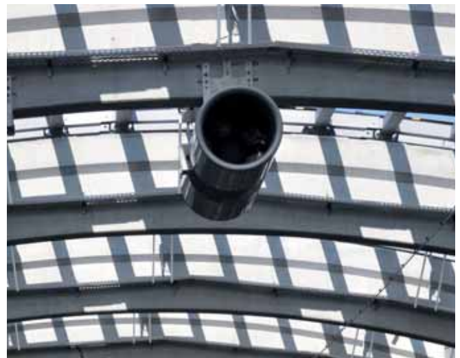
HTA 38/17 in HCR as attachment point for the ventilation units fixed to the precast concrete roof beams
