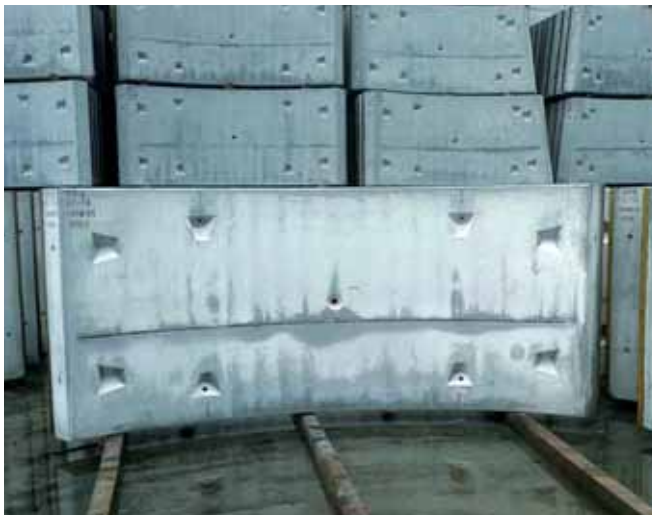
HALFEN HZA 29/20 Channels cast into tubbing segments
