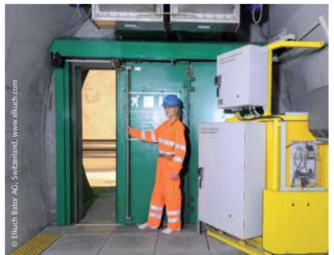
Installed sliding cross passage door, Gotthard Base Tunnel
