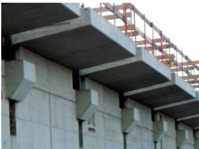
Using HSC elements to post-installed reinforced concrete corbels
