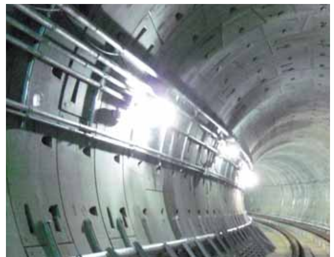
Fixing of pipe systems
