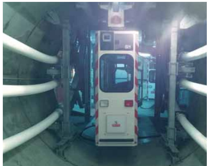
Overhead rail service car and heavy high power cables
