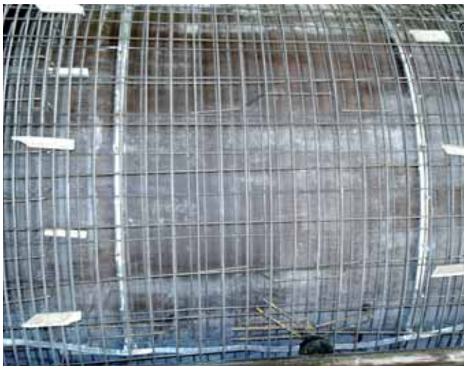
Reinforcement cage on steel formwork with serrated HALFEN channels
