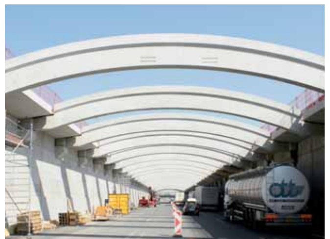
Supporting the prefabricated beams on the reinforced concrete corbels
