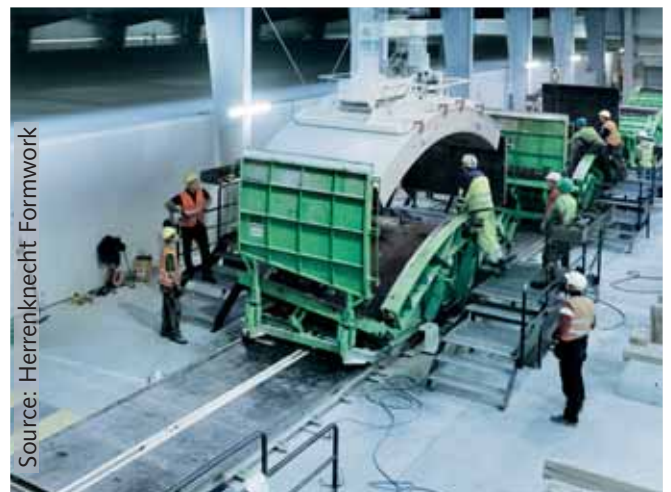
Lifting a tubing segment at a precast production plant
