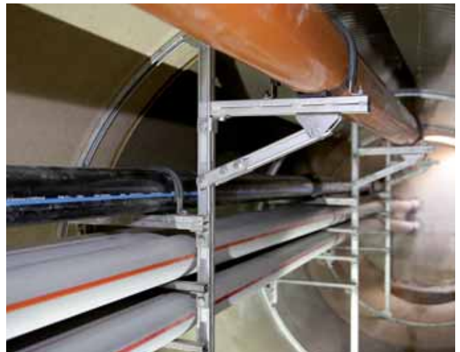
Sewer pipe support using brackets with pre-assembled fixings
