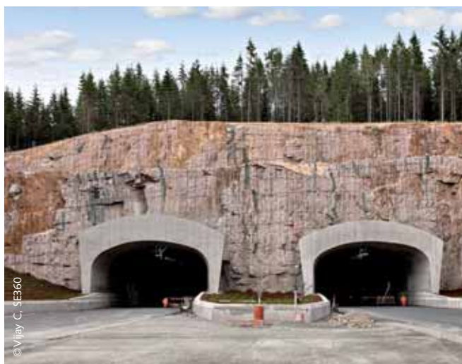
View of the tunnel approach, i.e. exit
