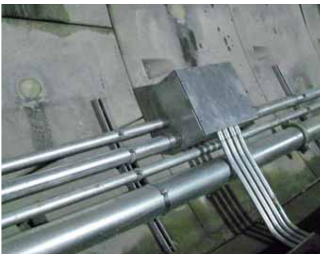
Fixing of pipe supports to galvanized, hot-rolled HM Channels
