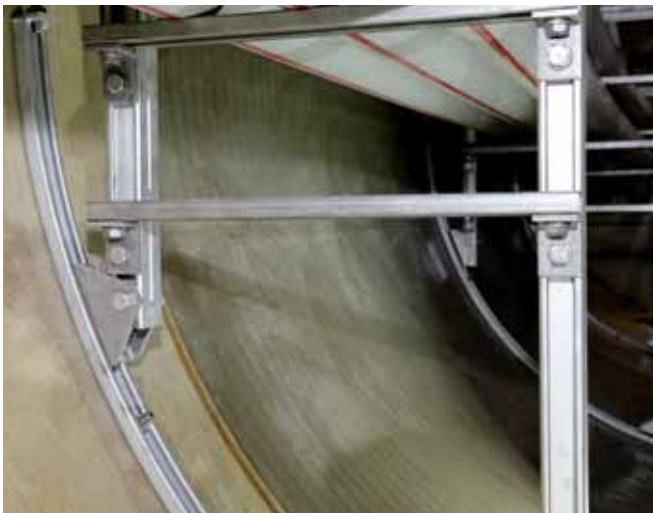
Round utility tunnel; service station, Switzerland Application: Powerclick System
