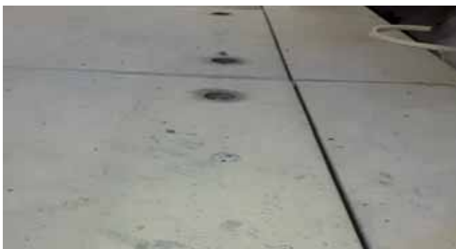
Cover slab; each slab has four cast-in KKT Spherical head transport anchor points
