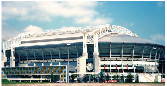
APPLICATION IN PRECAST ELEMENTS FOR STADIUMS
