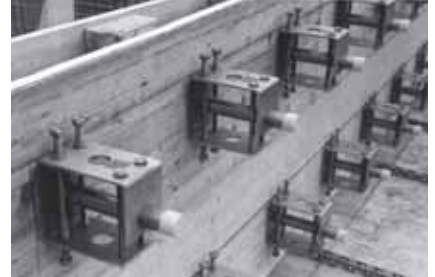
HSD-CRET sliding sockets nailed onto the formwork
